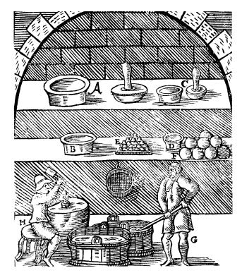
**FIGURE 9.** ■ Making cupels from calcined, crushed bones ground into a paste with beer and molded. The oxides of baser metals such as iron are absorbed into the cupel while molten gold or silver remain on its surface (Ercker, see Figure 5).
