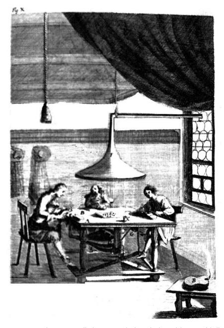
**FIGURE 158.** ■ Fabricating small glass toys with the aid of a pedal-operated bellows (from Kunckel's 1679 Ars *Vitraria Experimentalis*, from the Othmer Library, CHF).
